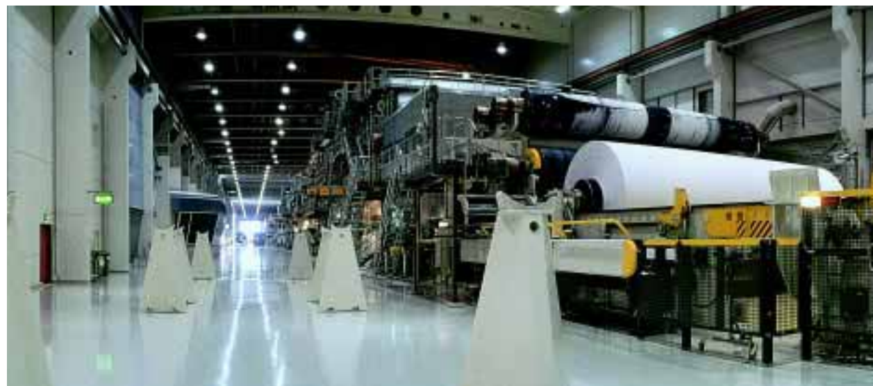
PPK7/PK7 machine hall, general view Stora Enso Oyj, Oulu, Finland
